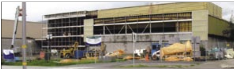
Above: Viking Construction: Kitimat Pool Project – August.
