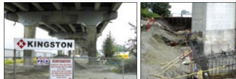
Kingston Construction at Knight Street Bridge (left) and Mitchell Island (right).
