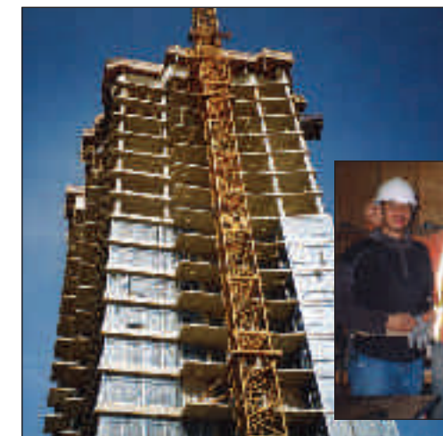
Left: Bosa's Persidia residential complex construction site White Rock, B.C.
