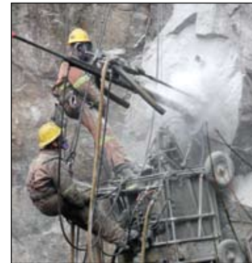
Capilano Suspension Bridge for the construction of an overhanging boardwalk, scalers Mike Talarico and James Haldane drilling and blowing out holes, and working off ropes and spider cage for rock bolting and anchoring to stabilize the cliff face.
