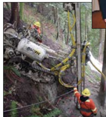
Members Peter Tazelaar operating the winch and brake while Joe Gauvin operates the airtrack controls at the Capilano Suspension Bridge.
