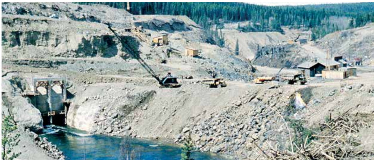
Kemano spillway. Photo courtesy of Rio Tinto
