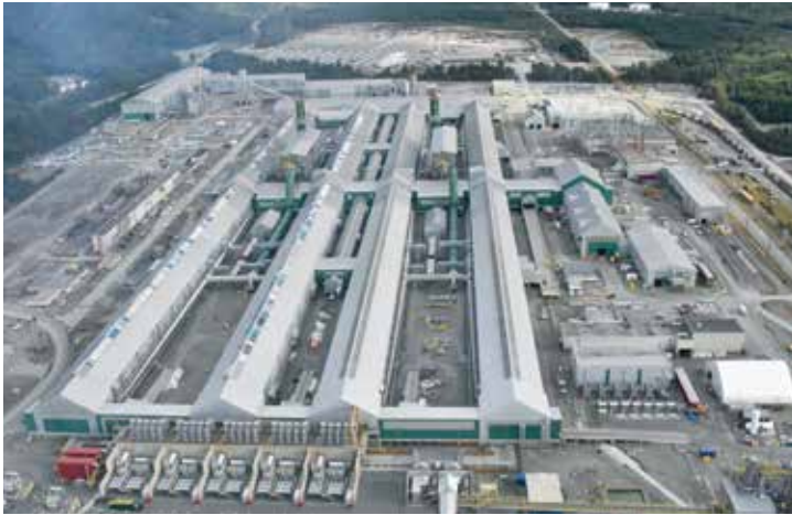
Completed Rio Tinto Modernization Project: Aluminum Smelter. Photo courtesy Rio Tinto
