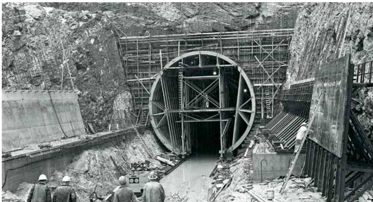
*Mica Dam tunnel outlet structure showing lining form in place.*
