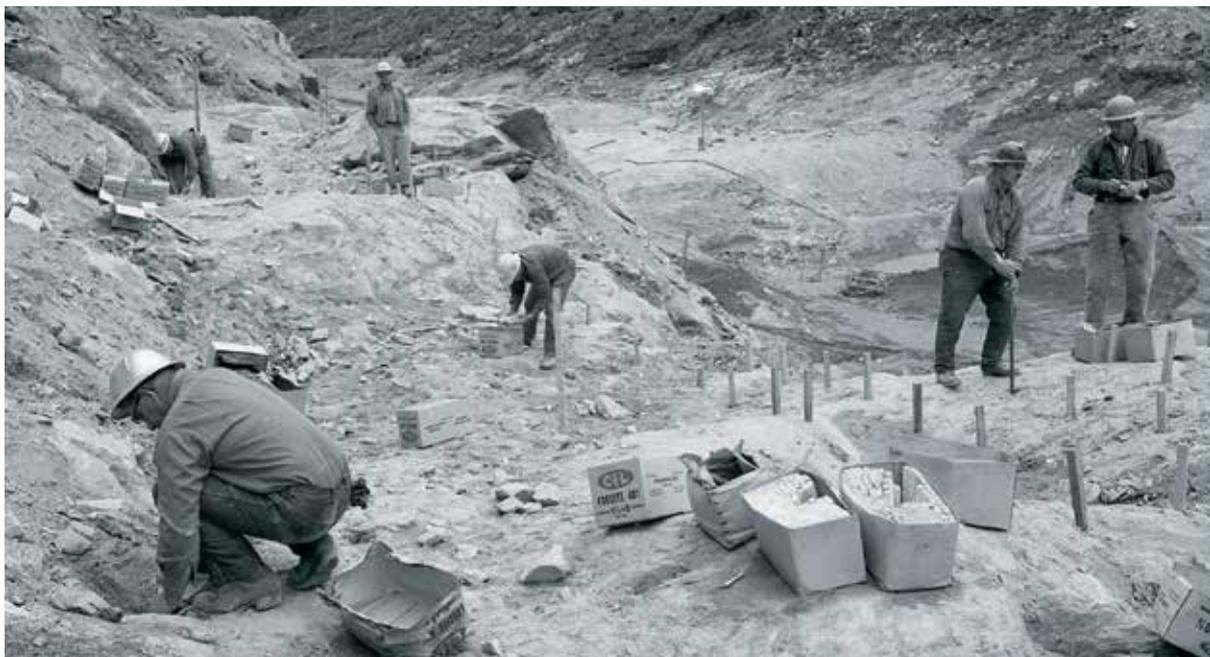
*Loading explosives on left abutment at Mica Dam.*
