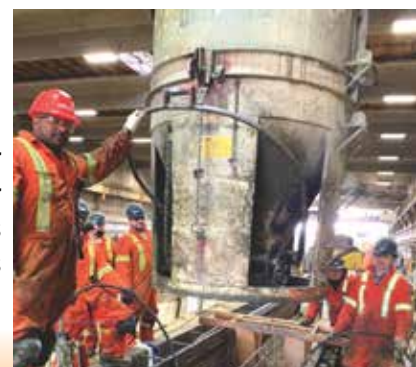
Members casting precast girders at Con-Force Structures
